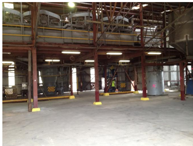
Piping being installed
