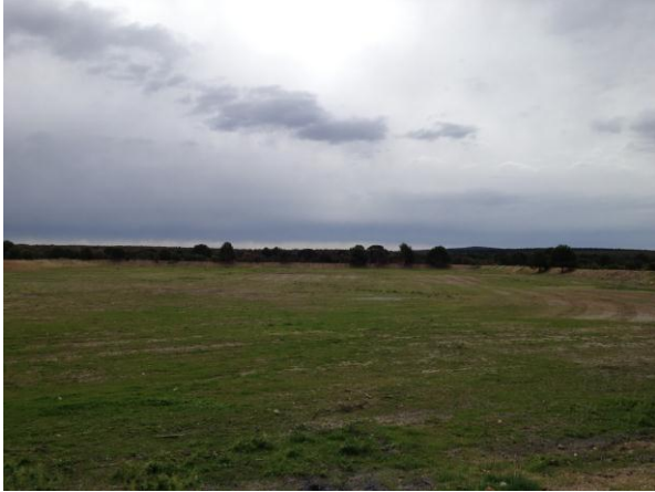
Tailings dam prepared
